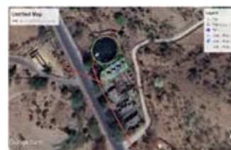
Water Treatment Plant
